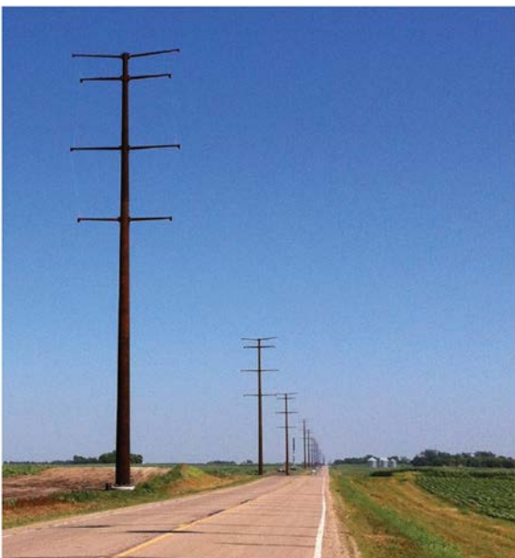
Single pole steel structures will primarily be used to reduce land impacts; some locations may require two pole structures. Poles are between 140 and 170 feet tall and will be about 1,000 feet apart. Typically, a 150-foot wide right-of-way will be required.
